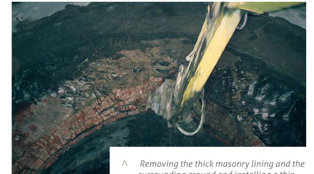
▲ Removing the thick masonry lining and the surrounding ground and installing a thin shotcrete shell.
