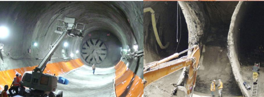
Beacon Hill Station is a deep-mined underground station located in complex glacial soils with multiple groundwater horizons. DSP was retained as a specialist consultant for the final design of the large NATM / SEM / SCL station tunnels, as well as various cross passages and adits.
