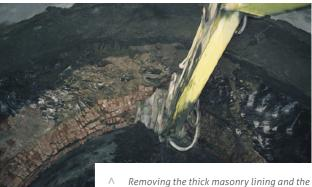
Removing the thick masonry lining and the surrounding ground and installing a thin shotcrete shell.
