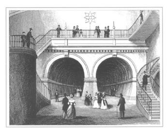
THE THAMES TUNNEL, constructed by Marc Brunel between 1825 and 1843, was the world's first bored tunnel river crossing. Originally designed for horse and foot traffic, the tunnel today is part of the London Overground transit system. Dr. Sauer & Partners designed the rehabilitation scheme and supervised the implementation of the re-profiling, shotcrete, and waterproofing works.
